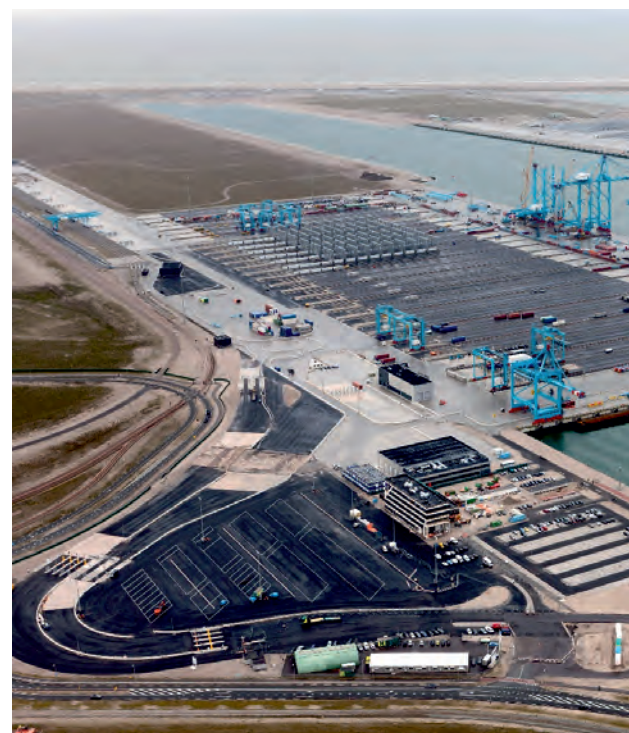
APM Terminal Maasvlakte II – Rotterdam, Niderlandy. APM Terminal Maasvlakte II - Rotterdam, Netherlands.
